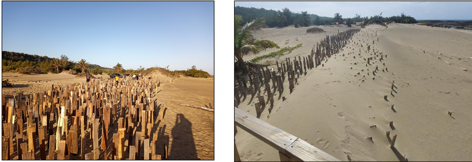
Figure 1. Biomimicry matrix on a breach on the primary dune in Secret Spot Beach, Isabela. The image on the left was taken on February 25, 2021 and the one on the right was taken on September 28, 2022. Note the large volume of sand accumulated on the mimicry. This was caused by the storm surge caused by hurricane Fiona on September 18, 2022.
