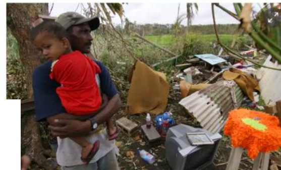
Fijian resident looks at the damage caused by Cyclone Winston . Photograph: AFP/Getty Images
