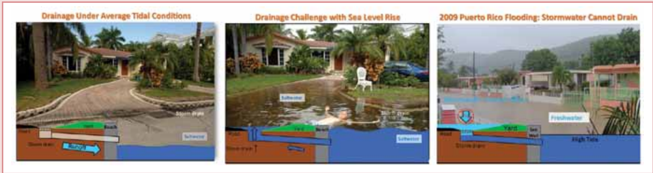
Figure 5 Gravity stormwater drainage under average tidal conditions, with sea level rise, and when combined with extreme precipitation events. (Photos 1 and 2 courtesy of the Broward County Government, Florida)
