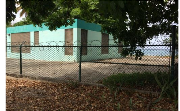
Wastewater Pumping Station
